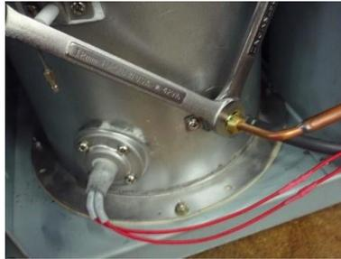
2. Use vice grips, locked onto the fuel nozzle in the upside-down position, as pictured. The nozzle enters the burner assembly at a downward angle. Positioning the vice grips like this will allow you to pull at the correct angle as the nozzle is removed, reducing your chances of bending the nozzle tube. Rotate the nozzle gently as you pull.
