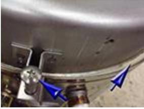
10. 1Wrap your shop-vac hose with rags/newspaper , insert into the burner throat, and turn the shop-vac on. This will keep the work area and your breathing air cleaner. Use of an N95 dust filter mask and gloves is recommended.
