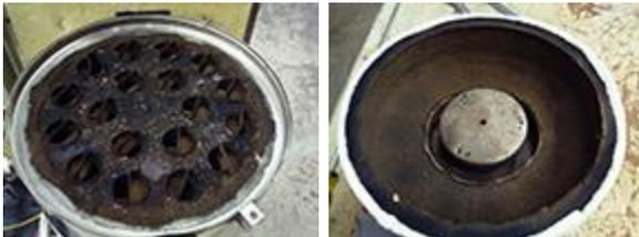
12. Cover the heat exchanger with newspaper or paper towels to increase suction in the tube you are working on. Securely grip the top of one of the baffles and use a gentle twisting and up/down motion to remove it. Longnose bent pliers work well for this.
