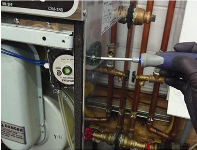
7. Remove the oil line section going between the fuel strainer and the fuel pump. (17mm on pump, 14mm on strainer, & 12mm on fuel line). Use a backup wrench as pictured.
